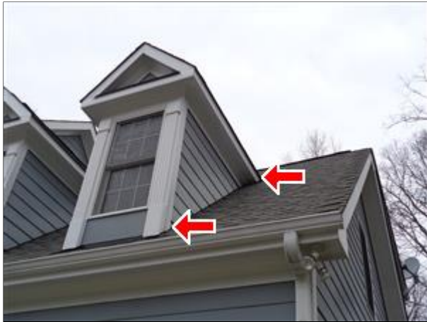
2.0 Picture 1 The right side of the right dormer.
