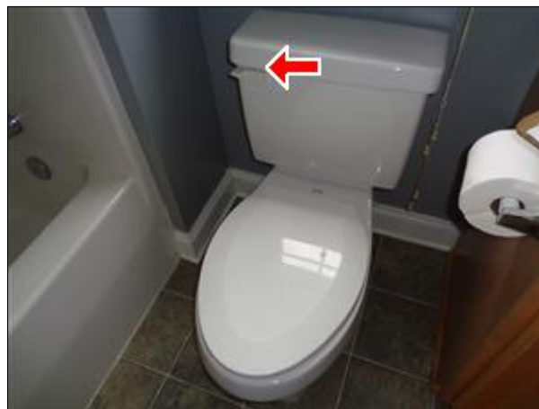
6.0 Picture 2 The commode in the hall bathroom upstairs.
