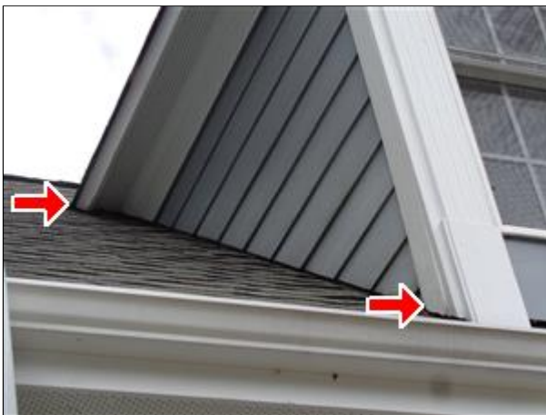
2.0 Picture 3 The left side of the right dormer.
