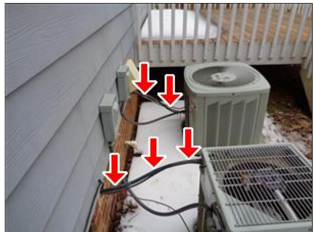
8.8 Picture 2 The lines without the coverings.
