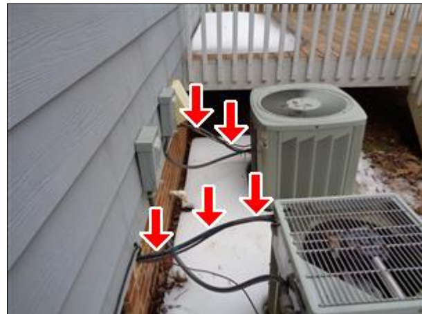
8.8 Picture 2 The lines without the coverings.
