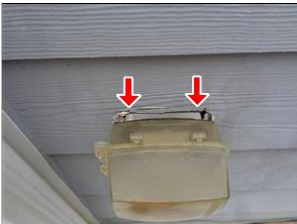
7.3 Picture 1 The electrical box on the back of the house.
