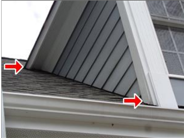
2.0 Picture 3 The left side of the right dormer.
